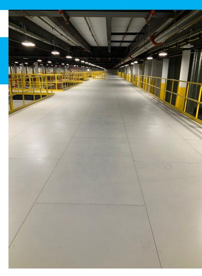
ResinDek flooring panels are backed by a 10-year product warranty and have proven structural integrity that supports live and dead load limits from 2,000 – 8,000 lbs. For more information email us at <a href="mailto:info@resindek.com">info@resindek.com</a>.
